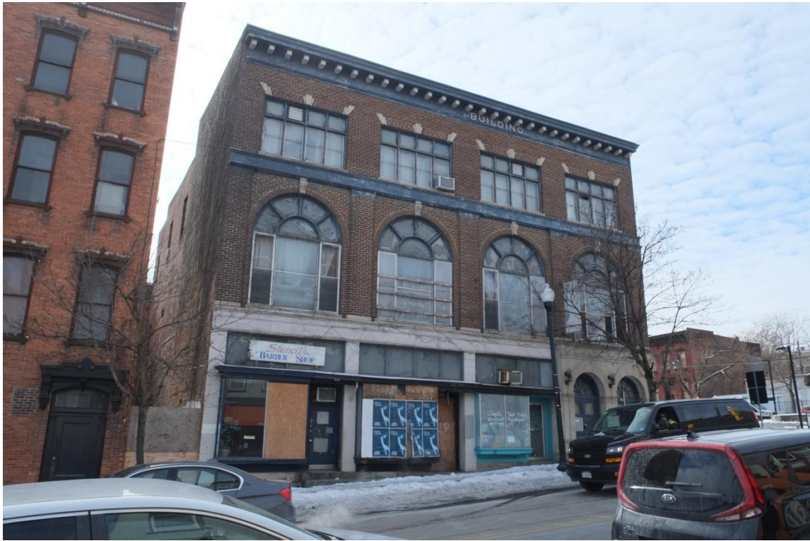
S-1: Primary (North) Façade, Facing SW
