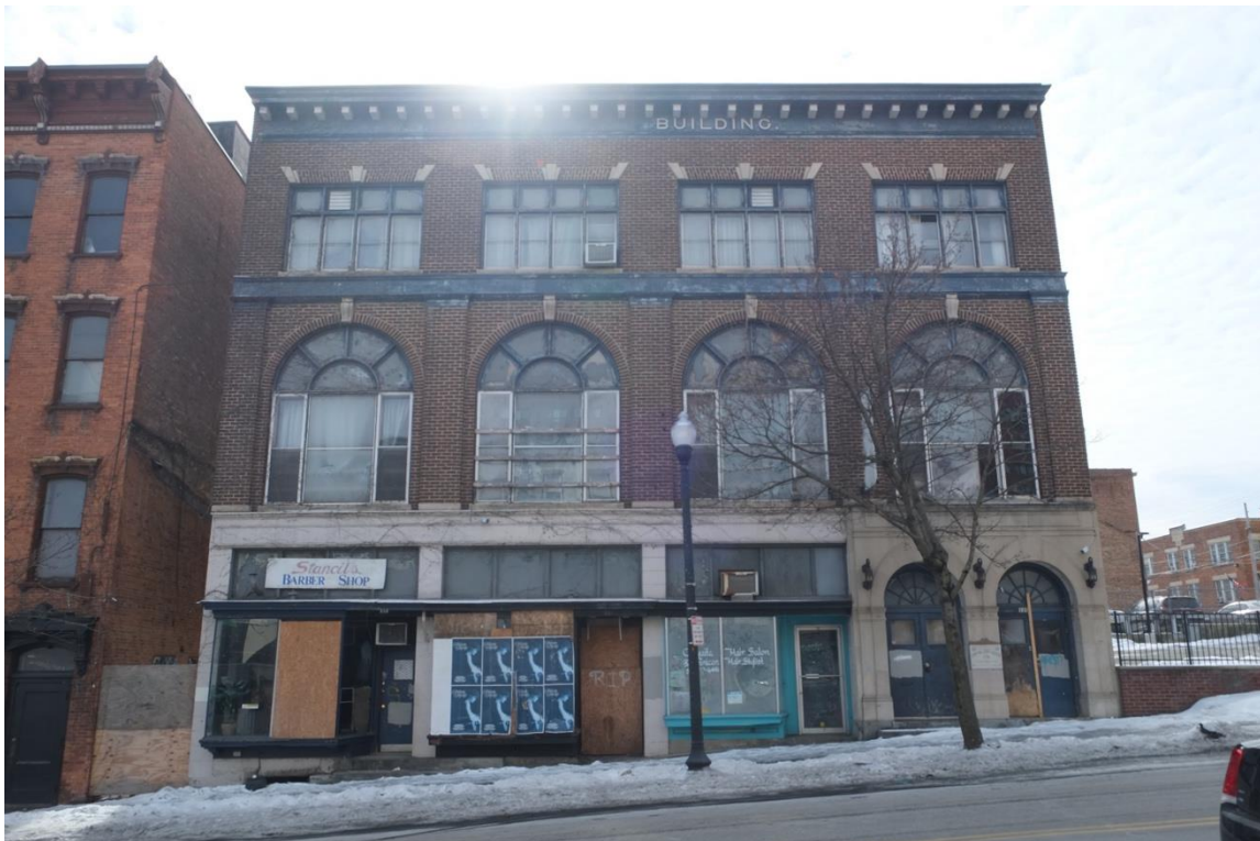
S-2: Primary (North) Façade, Facing S
