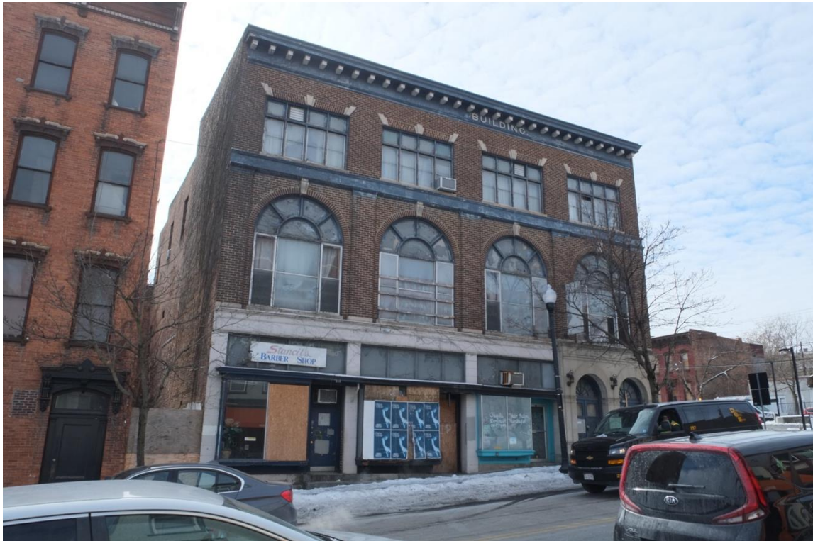
S-1: Primary (North) Façade, Facing SW
