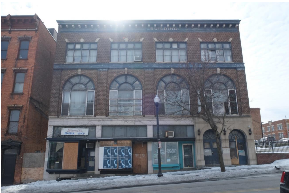
S-2: Primary (North) Façade, Facing S
