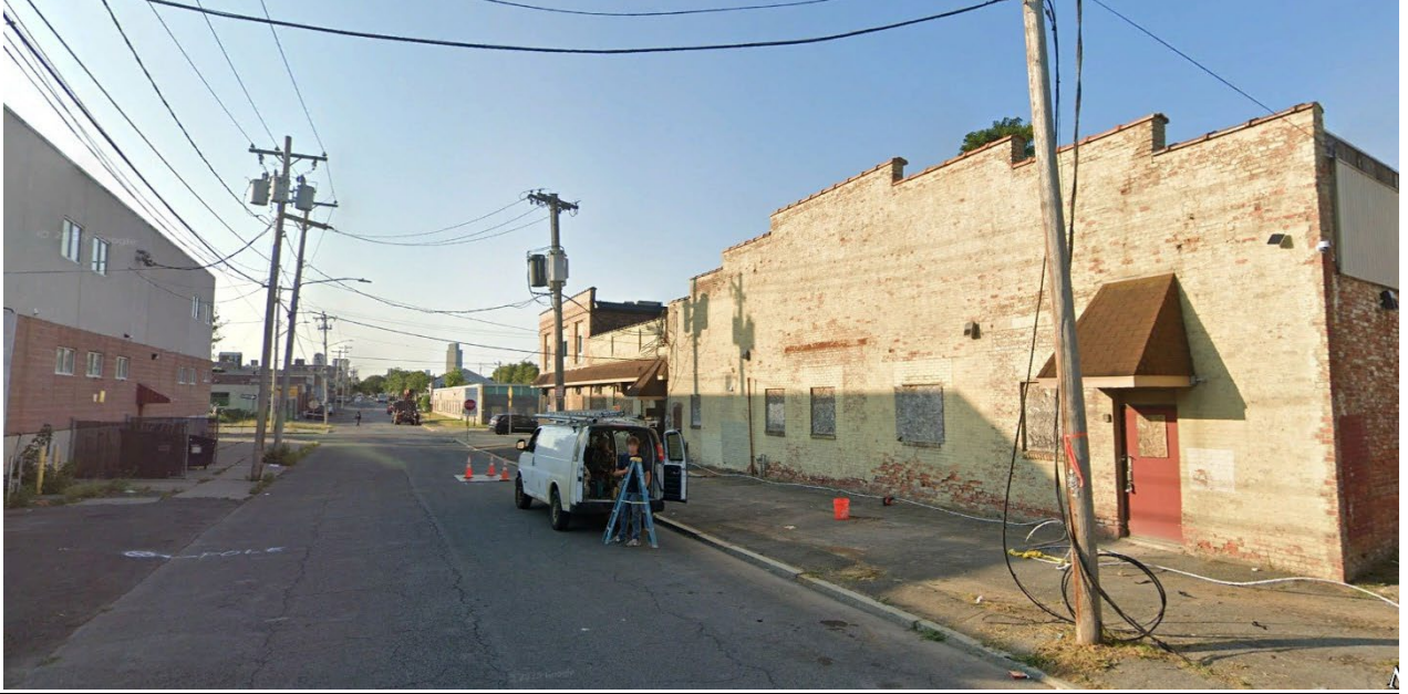
View from West end of building
