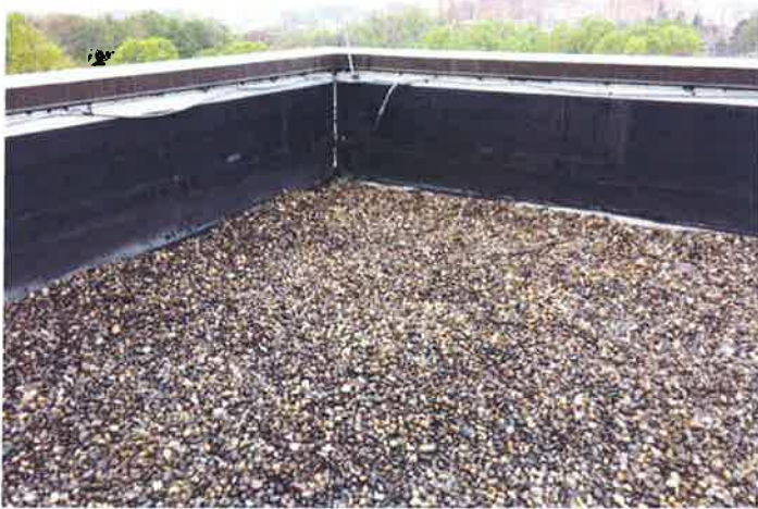
T 25 - Roof membrane is loose laid with stone ballast
