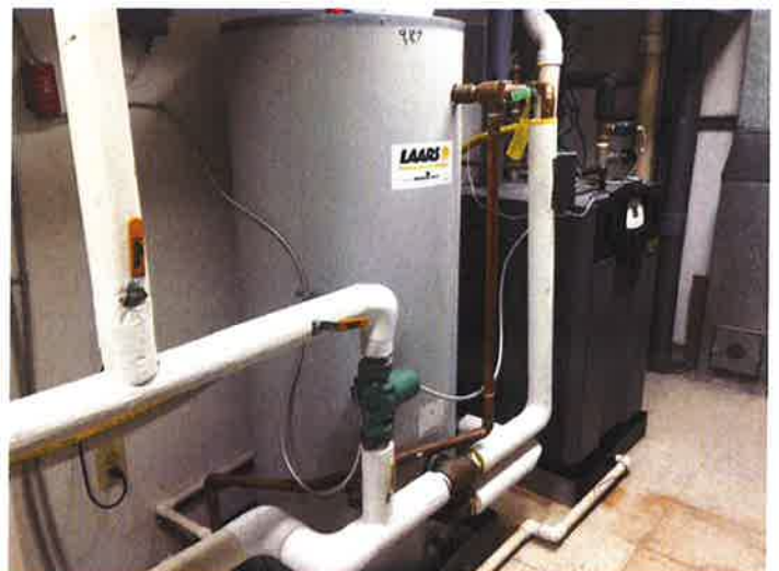
T 42 - Water heaters serve three floors
