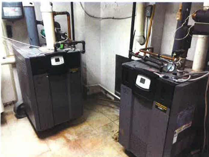
T 41 - Heating boilers serve two floors
