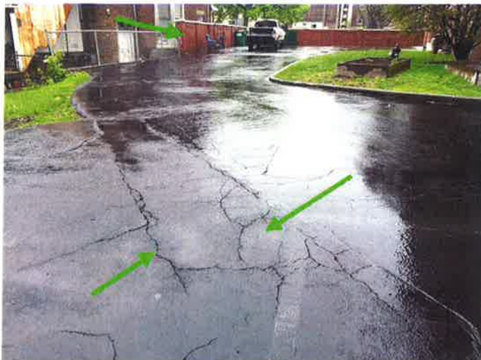
T 5 - Asphalt surface cracks
