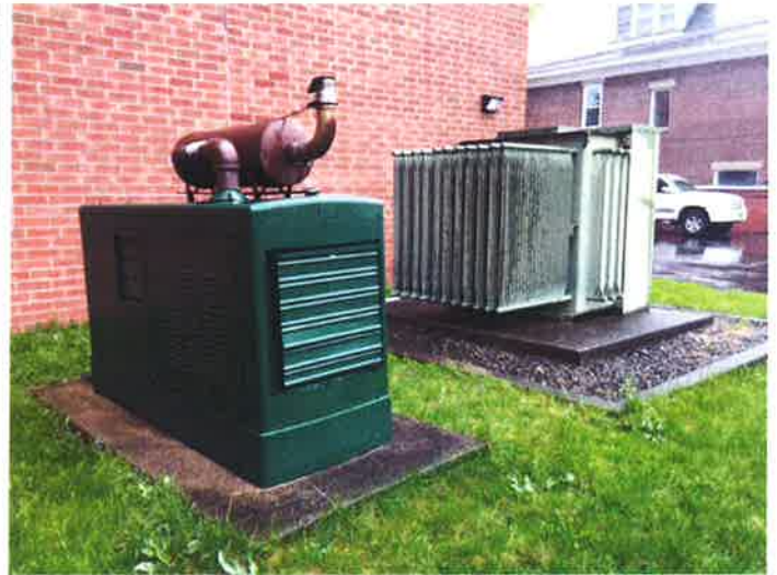
T 56 - Emergency generator and utility transformer
