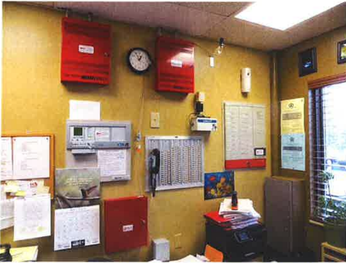
T 49 - Management office fire alarm and apartment communication panels
