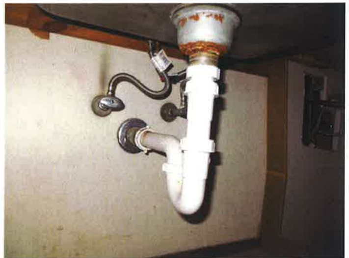
T 46 - Kitchen drains retrofitted with CPVS
