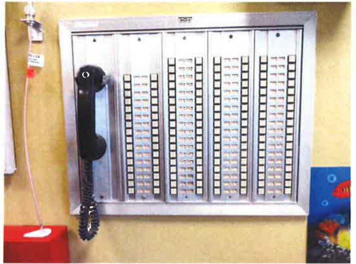
T 50 - Management office fire alarm panels
