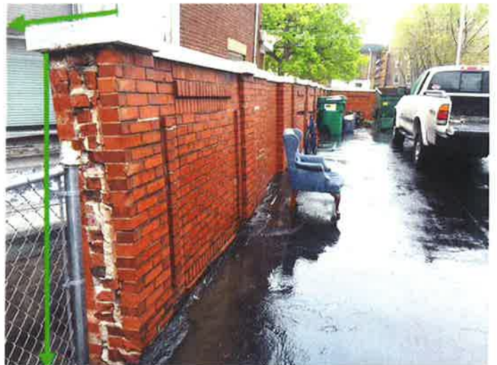
T 10 - Brick masonry wall leaning requires evaluation for repair
