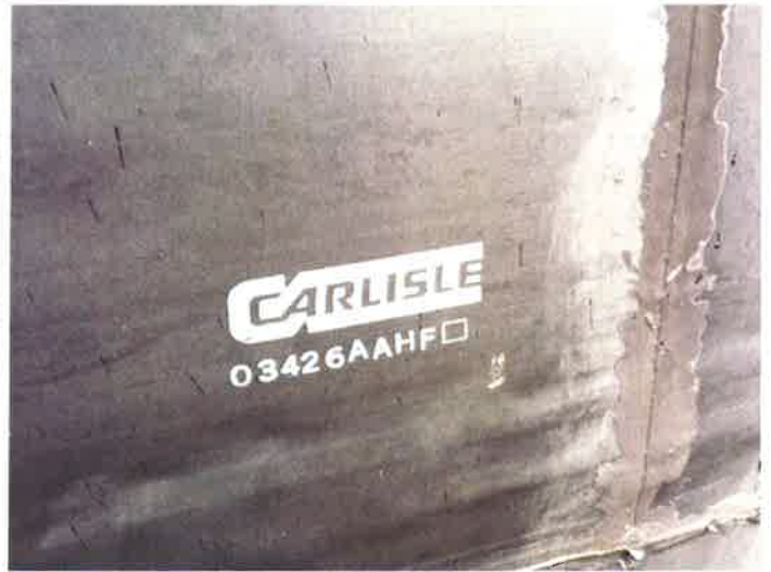
T 26 - EPDM single-ply membrane
