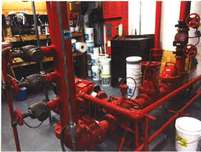
T 43 - Fire pump and sprinkler controls
