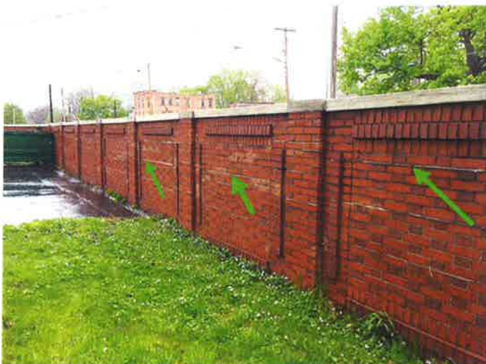
T 11 - Interior side of brick wall - tuckpointing is required
