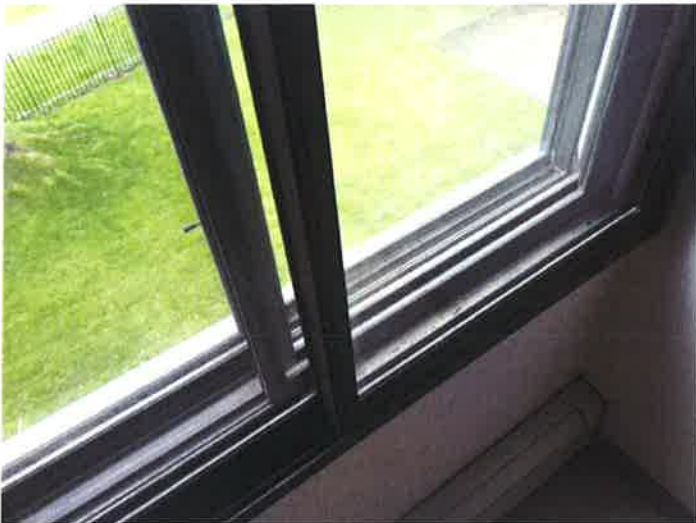
T 21 - Triple pane sliding window
