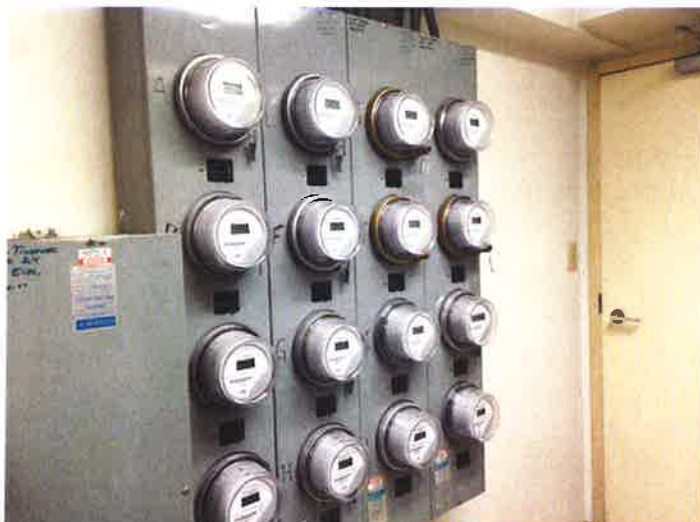
T 53 - Electric meter bank on upper floors
