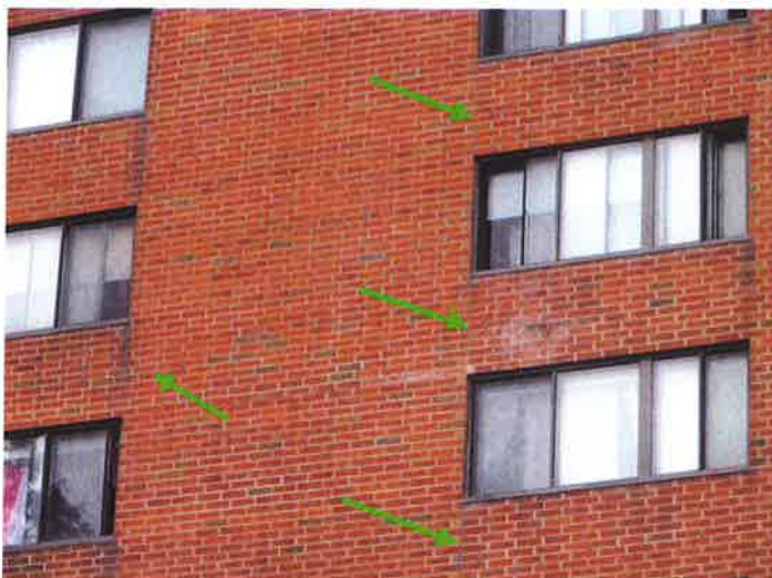
T 17 - Masonry control joint sealants have deteriorated
