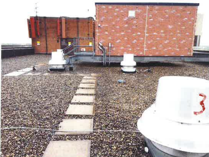
T 23 - Roof overview - exhaust fans
