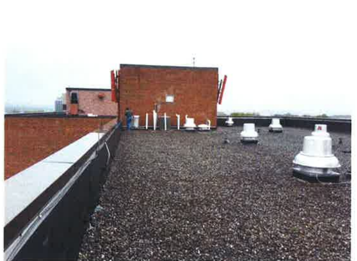
T 22 - Roof parapet wall with prefinished metal coping
