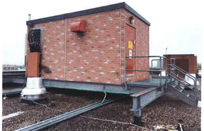
T 24 - Cellular equipment building sits on steel frame dunnage
