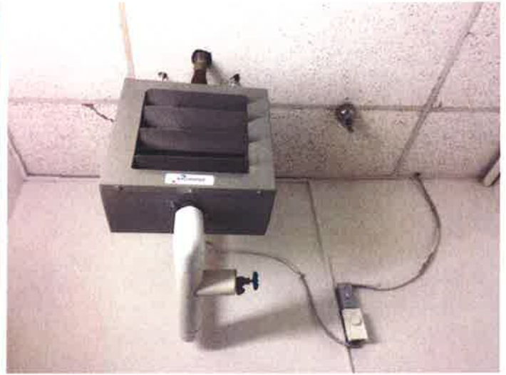
T 44 - Hot water supplied fan coil heater
