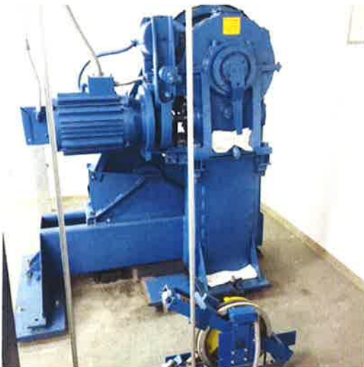
T 57 - One of two traction elevator motors
