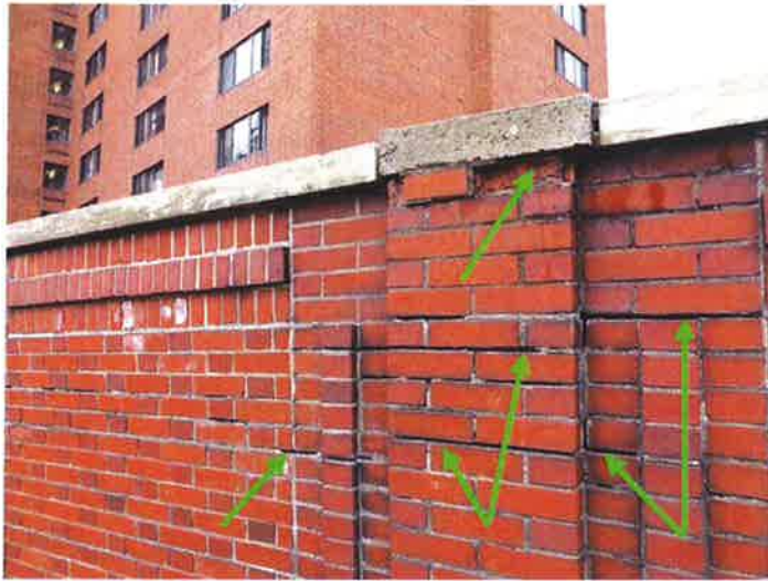
T 13 - Marble cap stone in good condition
