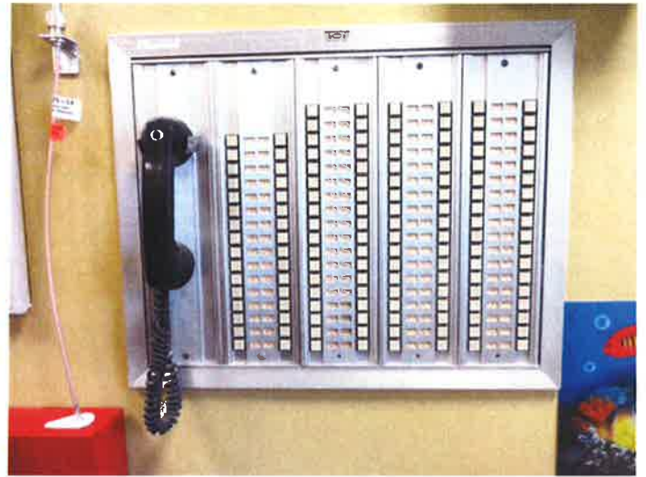
T 50 - Management office fire alarm panels
