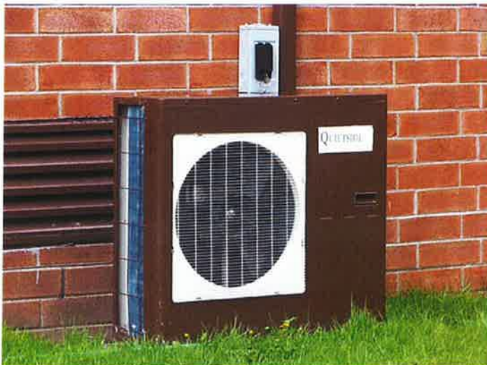
T 47 - Split system AC condensing unit
