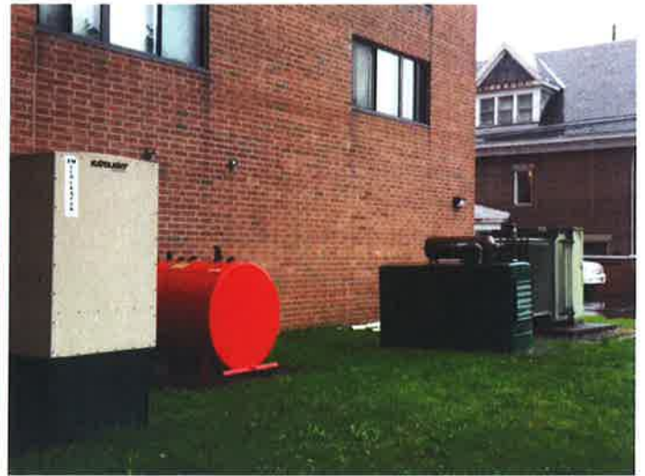
T 14 - Emergency generator and fuel tank
