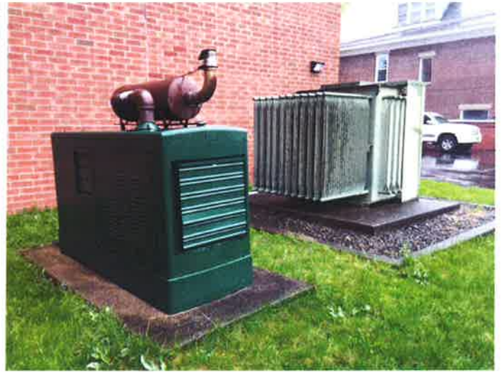
T 56 - Emergency generator and utility transformer
