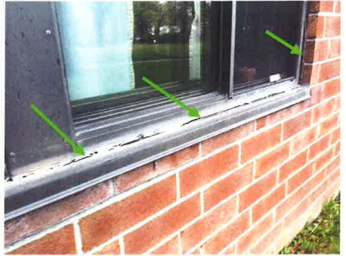
T 20 - Window frame joint sealants have deteriorated and require replacement
